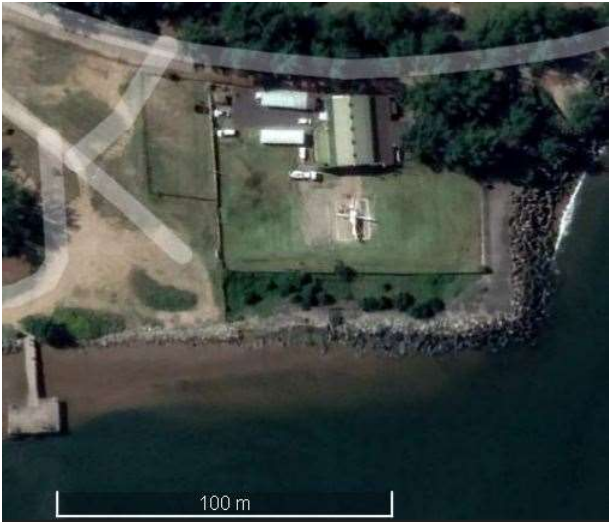
Figure 1.2 The current Helipad facility on the edge of the Richards Bay Estuary which is only able to accommodate two helicopters.
