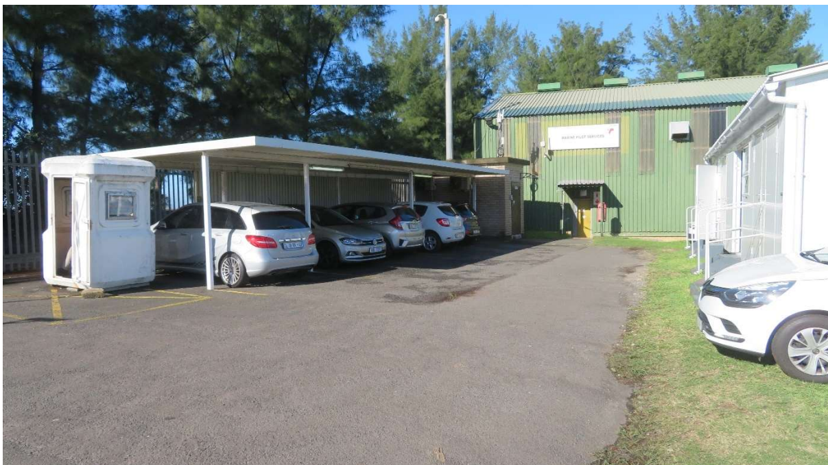
Figure 1.4 Car Park behind administration building and next to Helicopter hanger and workshop.
