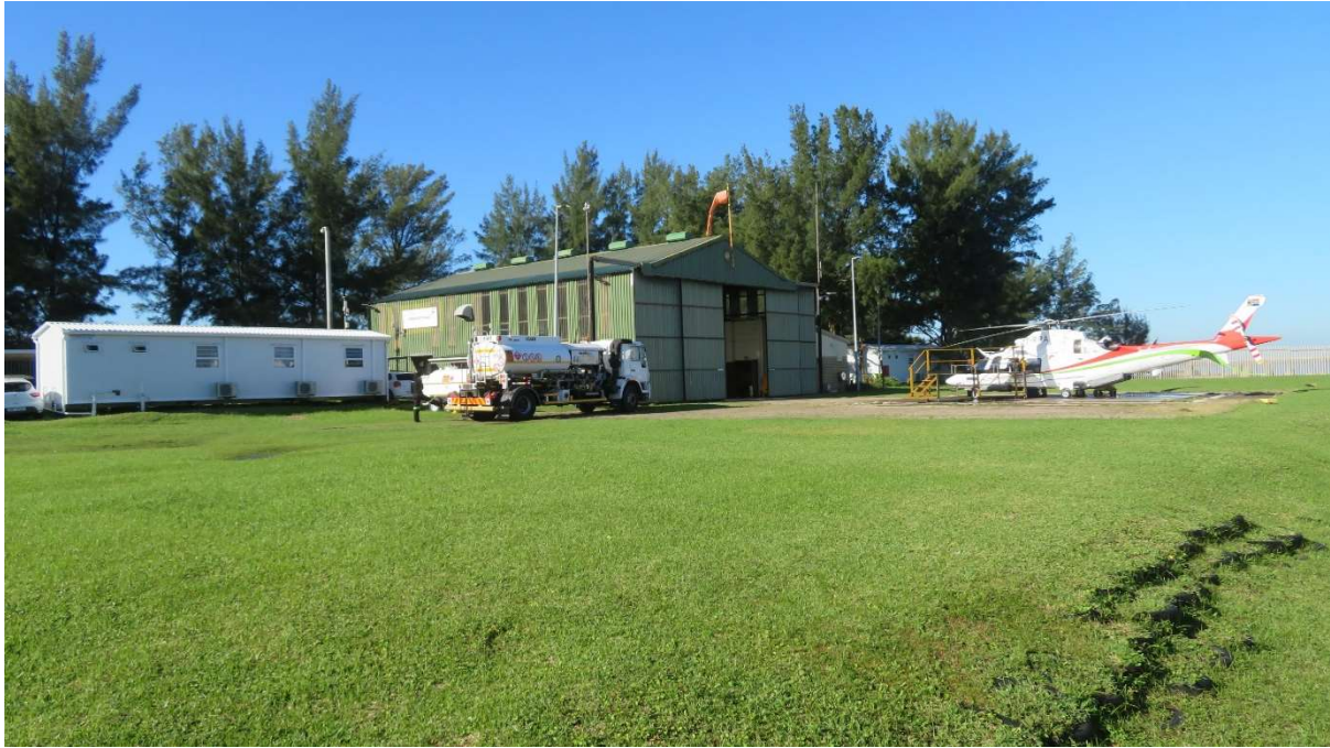
Figure 1.3 From right to left, Helicopter on Heliport landing platform, hanger and workshop containing second helicopter, refuelling tanker and administration building.
